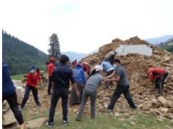
Removing the damaged materials of Stupa near Medical center
